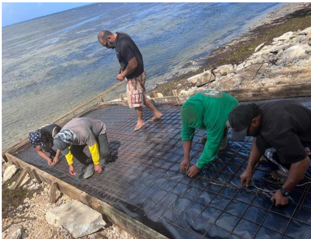
Repairing the boat ramp in front of Kanokupolu in 2023 after the 2022 tsunami
