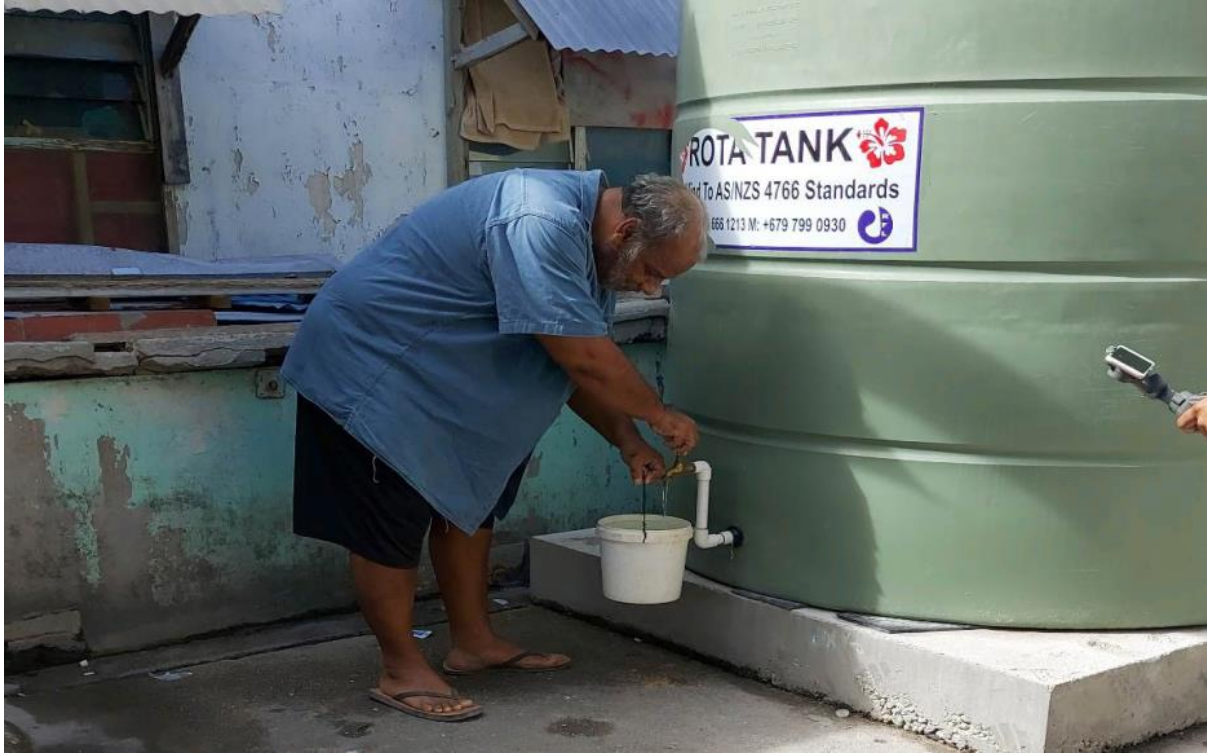
Resident fills a bucket from a tank provided by the project
