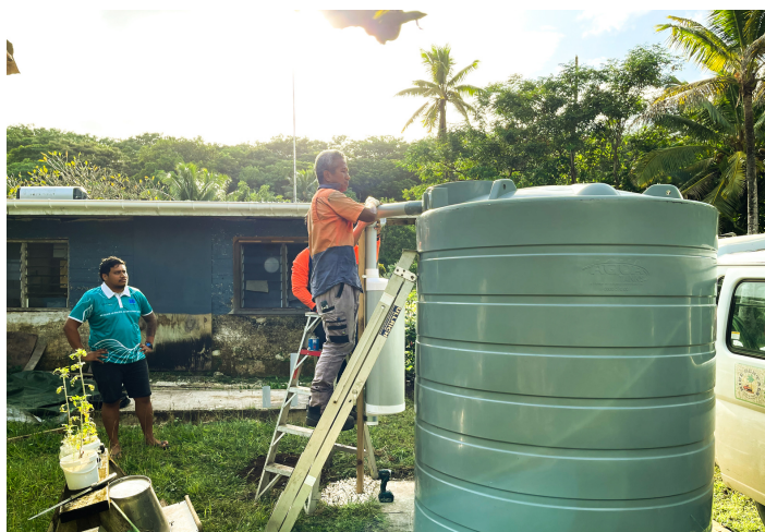
Project engineer connecting a tank to one of the selected houses
