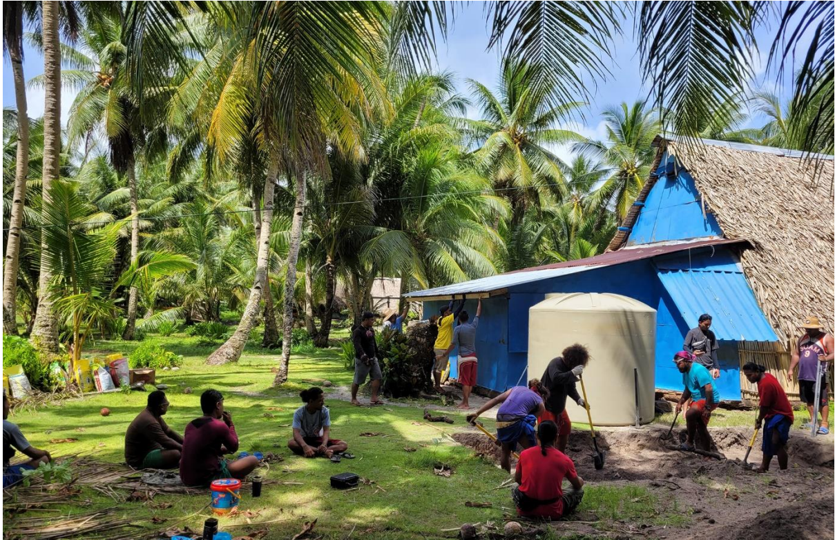
Community members helping with water storage tank installation at Pulusuk
