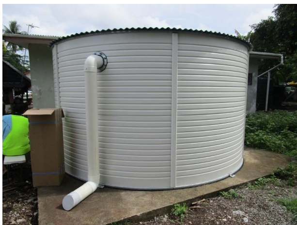
A Colorbond tank that was installed in Nauru
