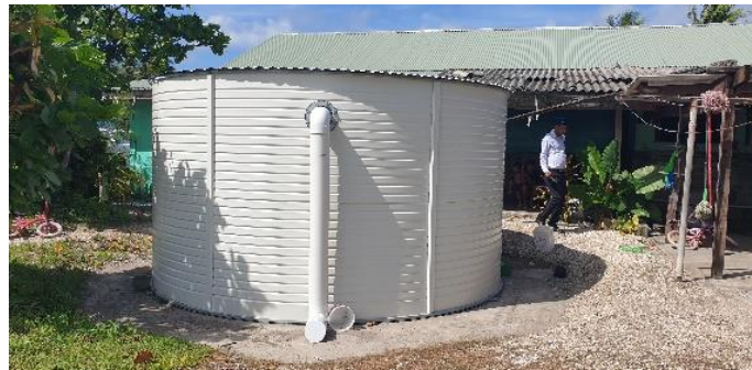
One of the Colorbond tanks installed by the Government of Italy
