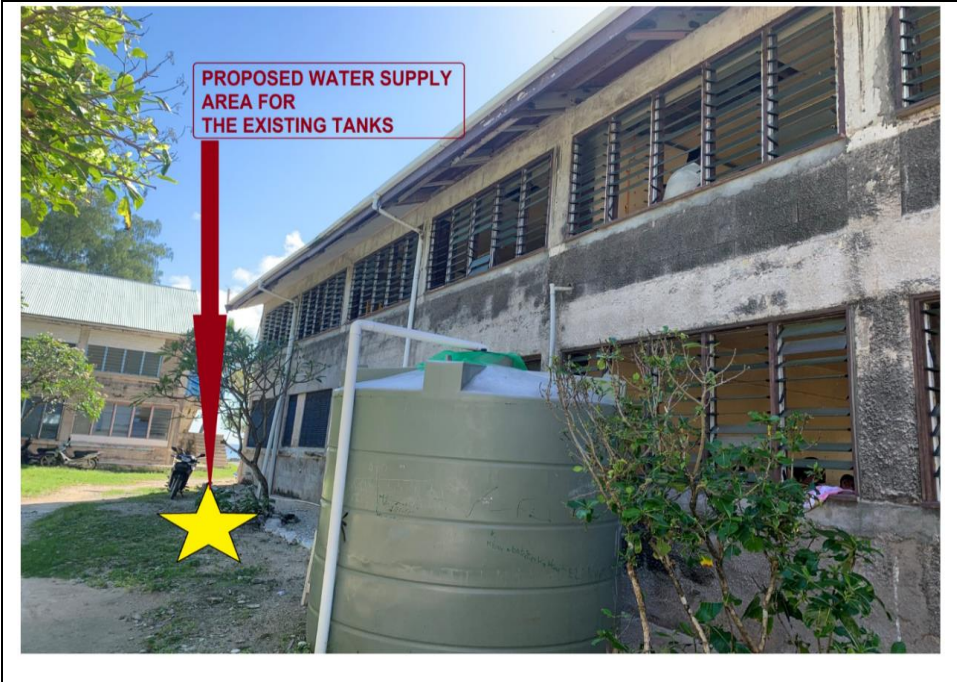
Photo # 3: View of the proposed location of the water supply area
