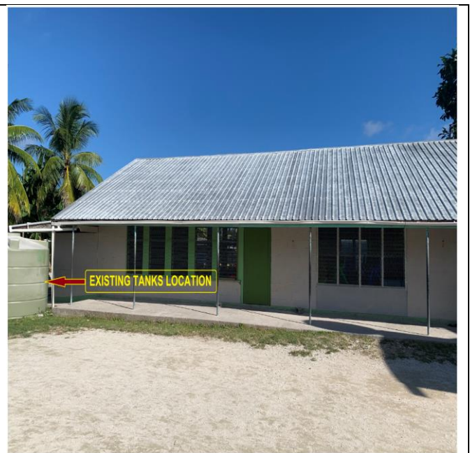
Photo # 5: Location of the existing tanks.
