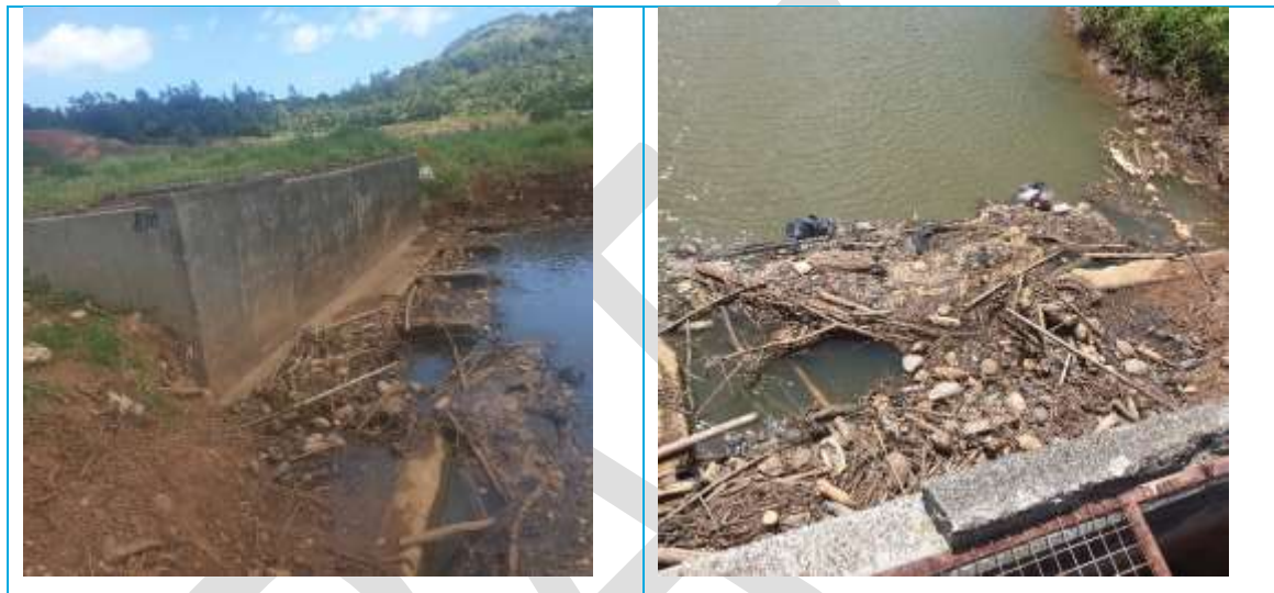
Figure 2-5: Levee and flood infrastructure at lower catchment (Source: Patrick Fong 2020)
