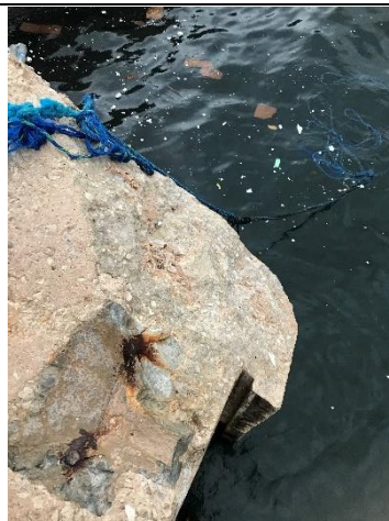
Fig A16 – Another jetty concrete structure 'chipped' at the end, one of the top corners. Damage measured length is 1.3m and 1m deep with 1.1m width.
