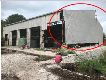
Fig A09 – leaning wall on the brink of collapsing.
