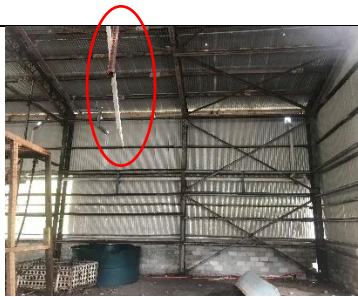
Fig A10 – Hanging sharp steel structures ready to fall anytime.
