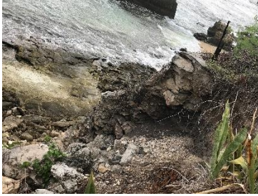
Fig A12 – view down the collapsed seawall 12m in length, roughly slightly more than 10m deep to the beach level. The collapse causes (what appears to be a) landslide.
