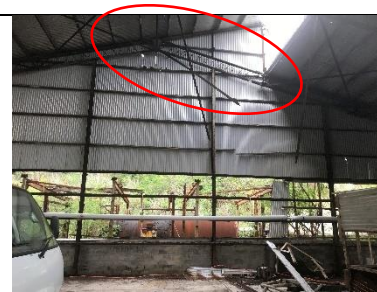
Fig A11 – snapped and disconnected steel ready to fall anytime.
