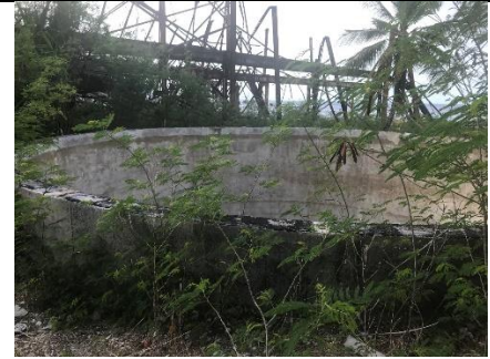
Fig A06 – Concrete tank reservoir, one of the two near the existing RO Shed (Cargo shed) with a collapsed roof.
