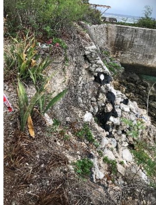
Fig A13 – view from the side at the top, same collapsed seawall.
